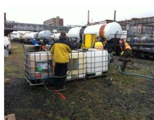
Test Injection of 3000 L of FeOx-NP in November 2014. Results are currently used for the preparation of the final remediation layout.
